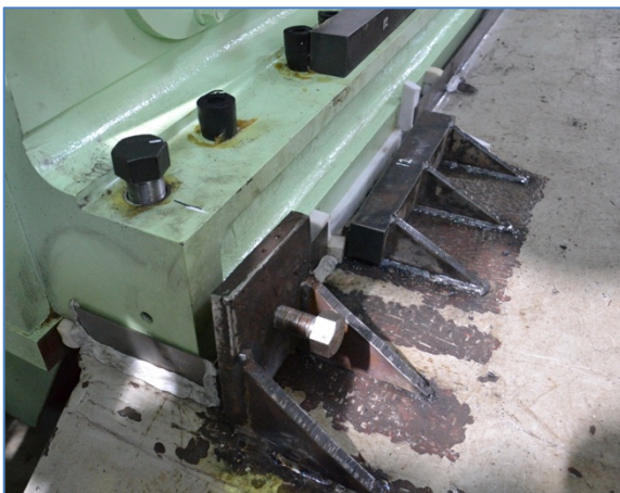
Figure 8: Damming and collision chock bracket installed prior to chocking
