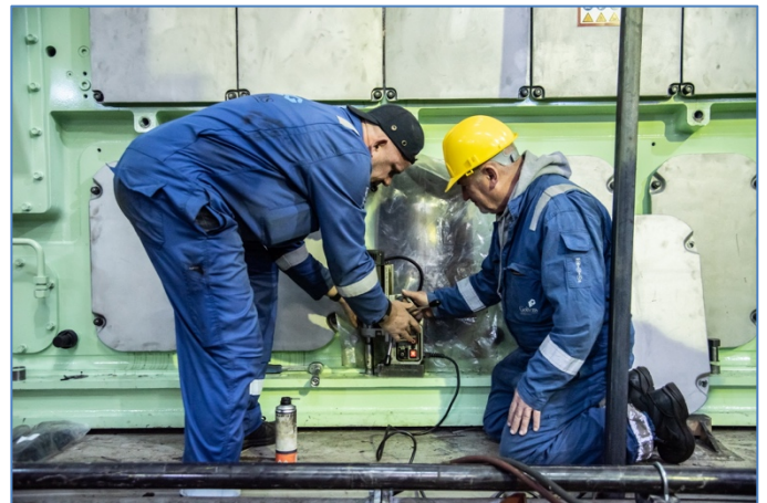
Figure 7: Preparing drill for foundation bolt drilling
