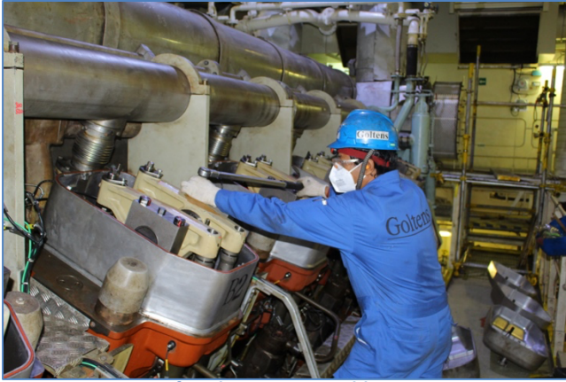
Figure 5: Torquing of Rocker Arm Assemblies
