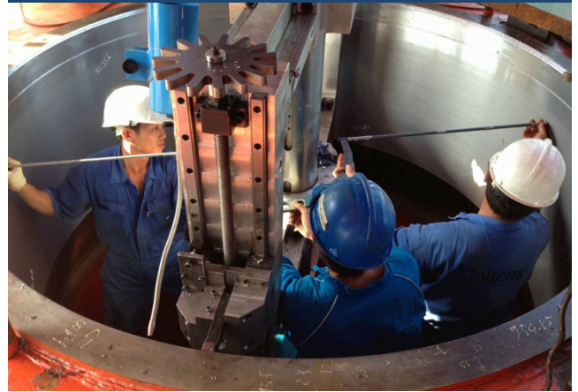
Checking of top bearing housing diameter
