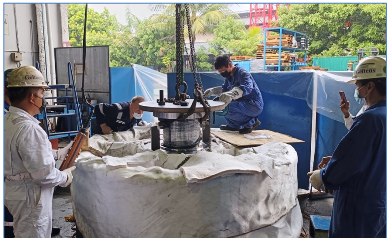
Installation of new Sprocket Shaft
