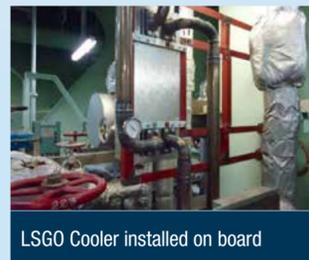
LSGO Cooler installed on board
