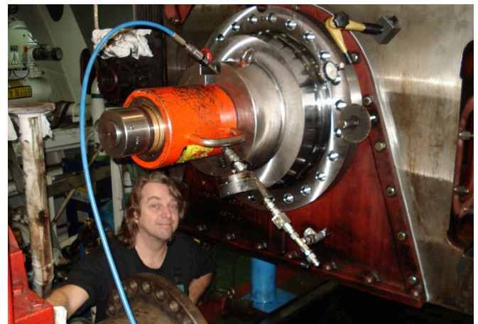
Preparing hydraulic installation of the flywheel hub
