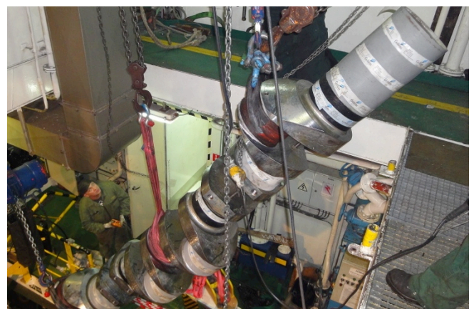
Rigging replacement crankshaft into the engine room
