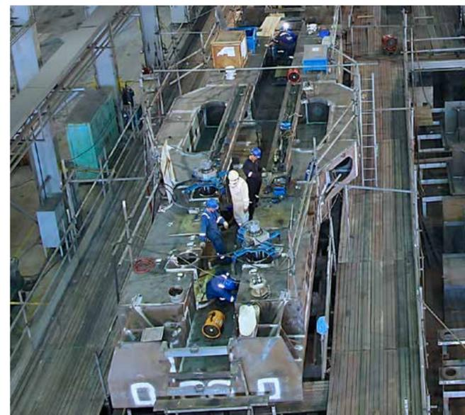
Boring equipment installed one of the six jack case structures for TAM DAO 5
