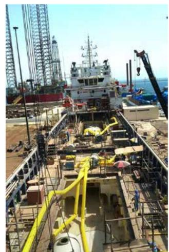
Tank install in process after compartment sealed with acid resistant coating
