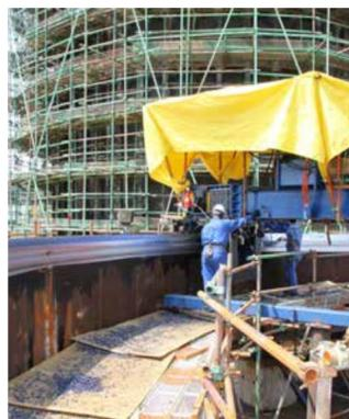
Machining top inside diameter at 5.2°
