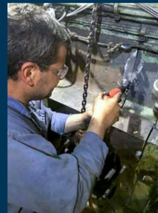
Drilling holes for stitch inserts along seam
