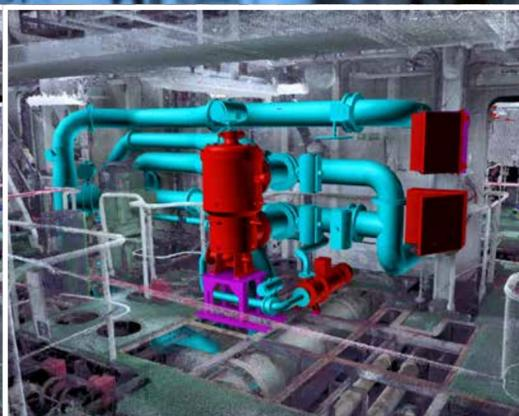
**3** The next step is to model the BWTS into the rendered room. At this point, it becomes possible to see exactly how the system would fit, evaluate rigging restrictions, locate power supplies and determine whether there will be sufficient space to walk around the system and service it.
