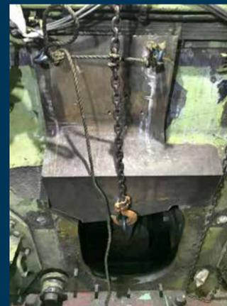
Cast and milled insert rigged into position
