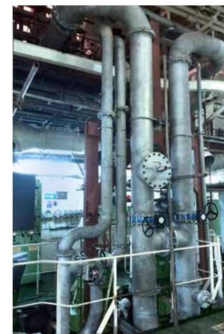
A portion of the BIO-UV Bio-Sea ballast water treatment system installed on a container ship
