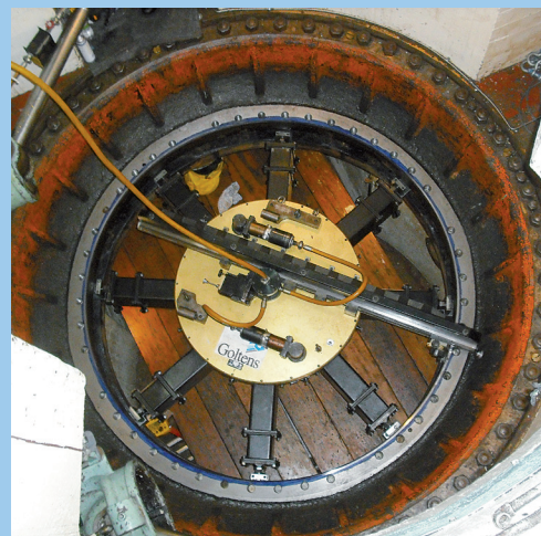
The in-situ machining of the foundation of a hydro-generator.
