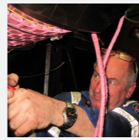
Installation of ceramic tile heating blankets for annealing
