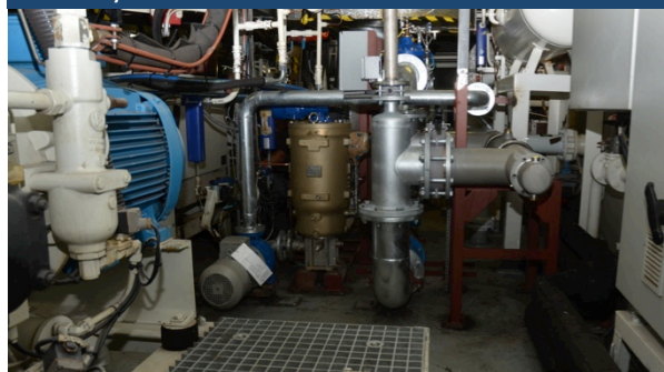
BWT system section after installation
