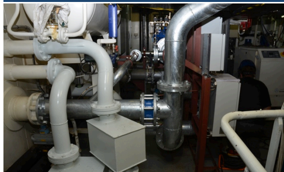
Section of BWT system after installation
