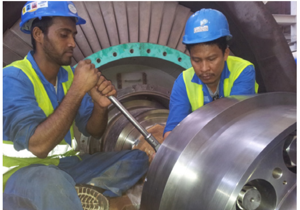
Goltens Saudi was engaged to perform in-place machining on six 1.2 meter diameter flanges on the gas lines connecting the SGT6-5000 gas turbines and reaming of the 114 turbine coupling bolt holes on six SST6-4000 steam turbines to bring the connections to required tolerances prior to connection at Qurayyah Power Independent Power Plant (QIPP). After completion, QIPP will be the largest combined cycle, gas-fired power plant in the world. The plant, located in the Eastern Province of Saudi Arabia, will generate ~4,000MW of power to feed the rapidly increasing power demands in the Kingdom.
