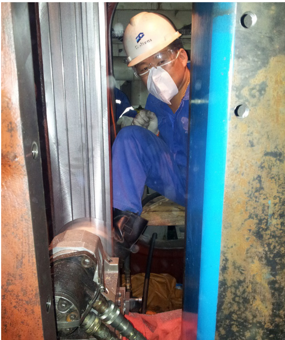
Goltens' In-situ Machining technician monitoring the progress of the guide rail machining on damaged Mitsubishi 6UEC52LA. Note deep vertical scoring on rails.
