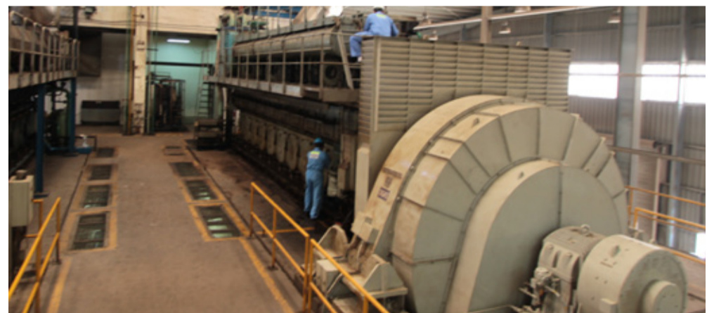
Goltens Diesel Technicians finalize work on one of the MAN B&W 9L58/64 engines at Star Cement.
