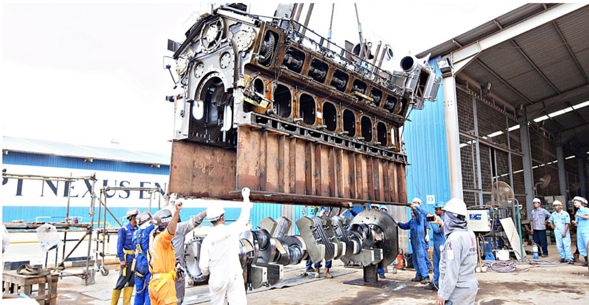
MAN B&W 12V32/40 engine block being rigged into place for the installation of the crankshaft after engine lineboring.
