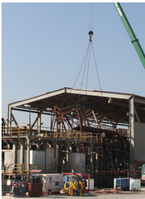
Work starts immediately to carefully remove the remnants of the burnt-out Accommodation Block, an exercise that took 3 weeks to safely complete before refurbishment work could progress.
