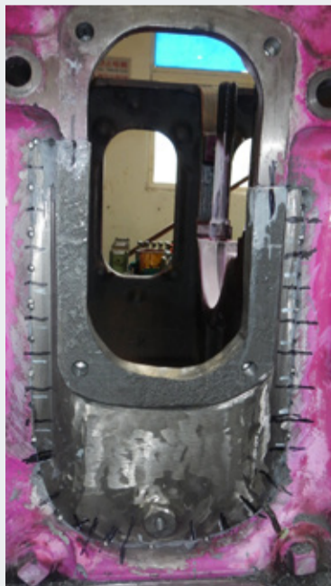
Pre-finish machining metal stitch repair. Full repair completed in only five days by Goltens Shanghai.
