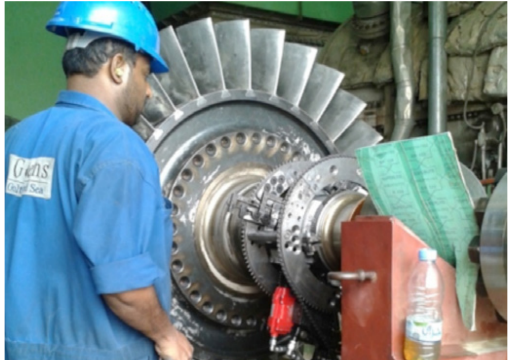
Saudi Electric Company (SEC) contacted Goltens Red Sea (Saudi) about damage to the shaft on a Fiat TG 20 B-7/8 Gas Turbine at their Narjan Power Plant. As the damage on the compressor bearing journal was more significant, Goltens' In-Situ machinists needed perform fine grinding and honing on the journal to remove the heavy scoring. Goltens removed the scoring taking only 0.25mm from the shaft diameter. As the damage to the exhaust side was less severe, Goltens was able to remove the lighter scoring with only honing and machine polishing.
