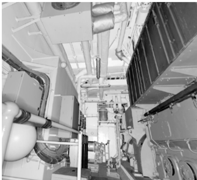
3-D scan and BWTS survey was carried out on board Coral Methane in 2013.
