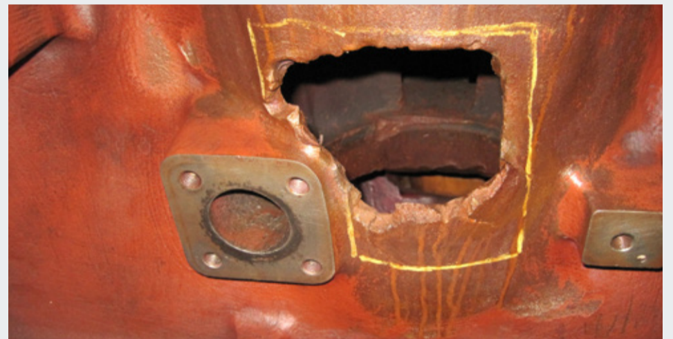
Damage resulting from a connecting rod failure on the vessel's MaK 12M282 engine.
