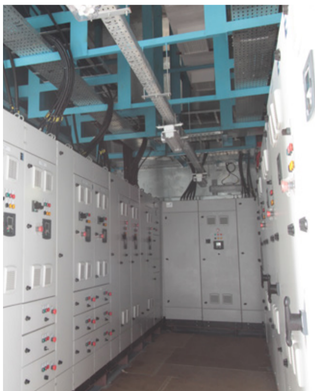
One of 6 MCC Panels in the MCC Room as part of a major electrical installation that also included PLC Cabinets, a SCADA System, and 32,000 metres of cable.
