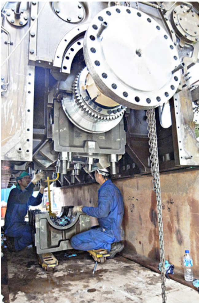
Installation of main bearings on the engine prior to rigging back on board.
