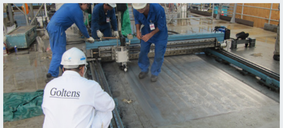
Flange facing of the underside of a turret head on an FPSO conversion project in Keppel Shipyard in Singapore (OD 5.99m/ID 5.58m)
