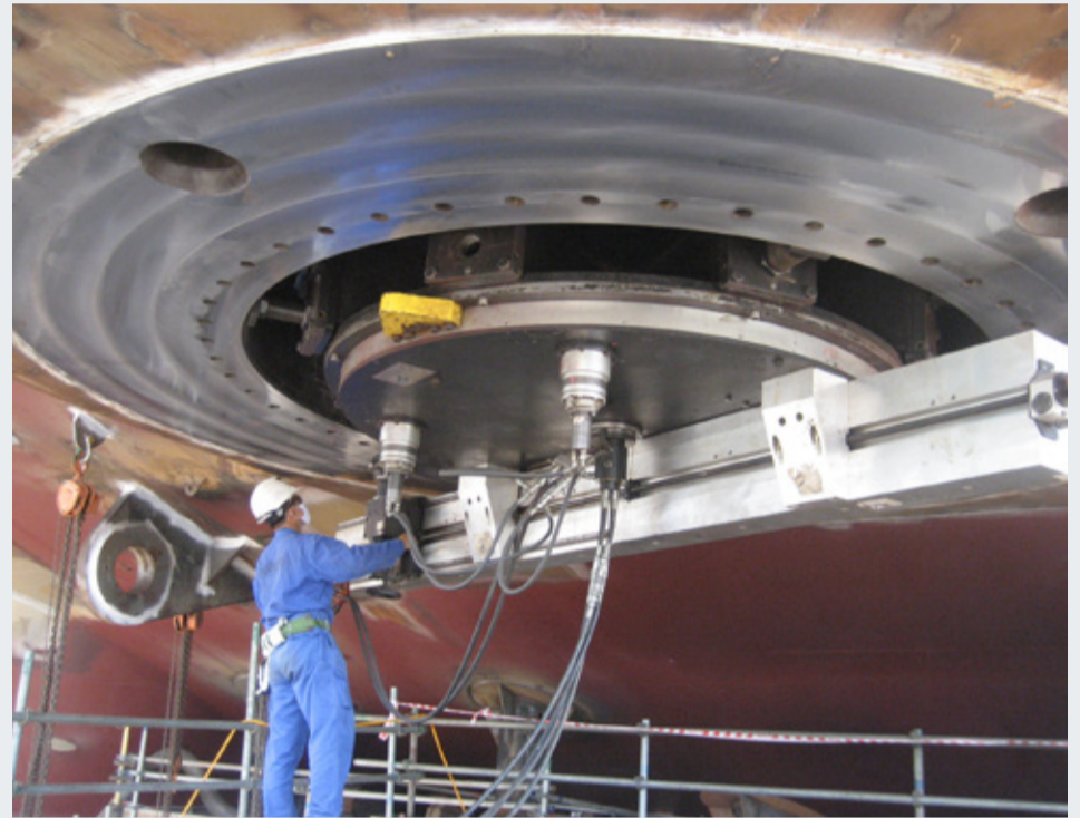
Goltens 6000i flange facing machine mounted on the 4.7m diameter flanges for the vessel's two 6MW Stern Thrusters. Machining was complicated by the inverted mounting of the machinery and the tight flatness tolerances of 0.15mm across the surface.
