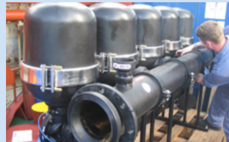
Goltens' technician preparing the Hyde Guardian filters for rigging into place in the engineering spaces.
