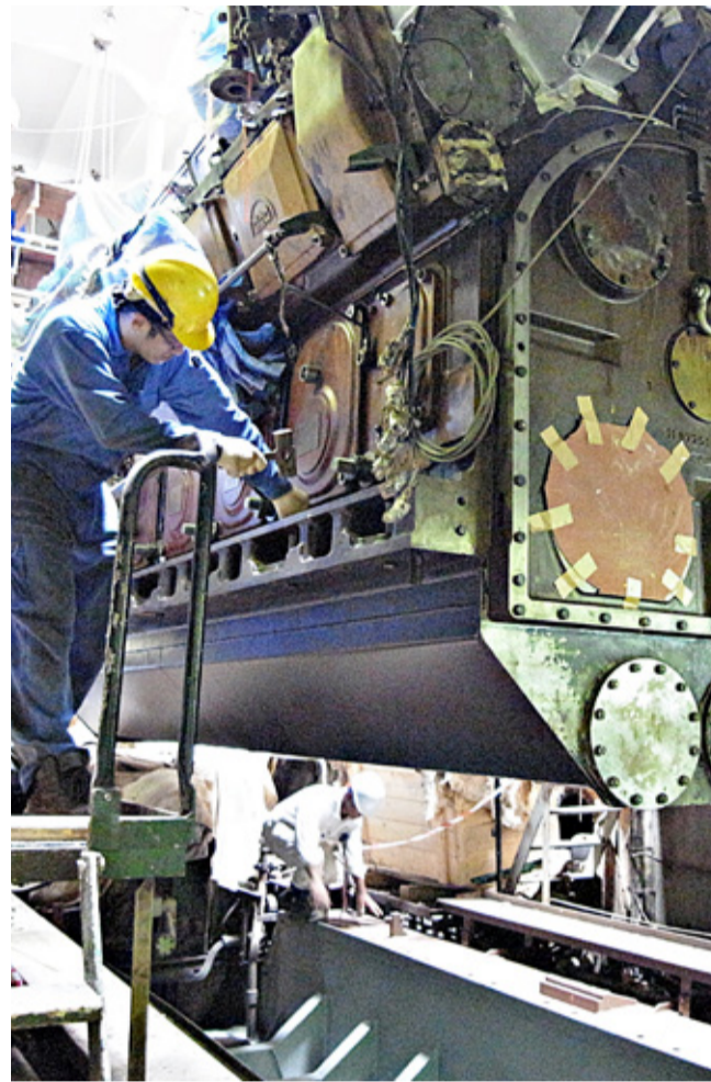
Lowering the repaired MAN B&W 12V32/40 engine into position in the engine room.
