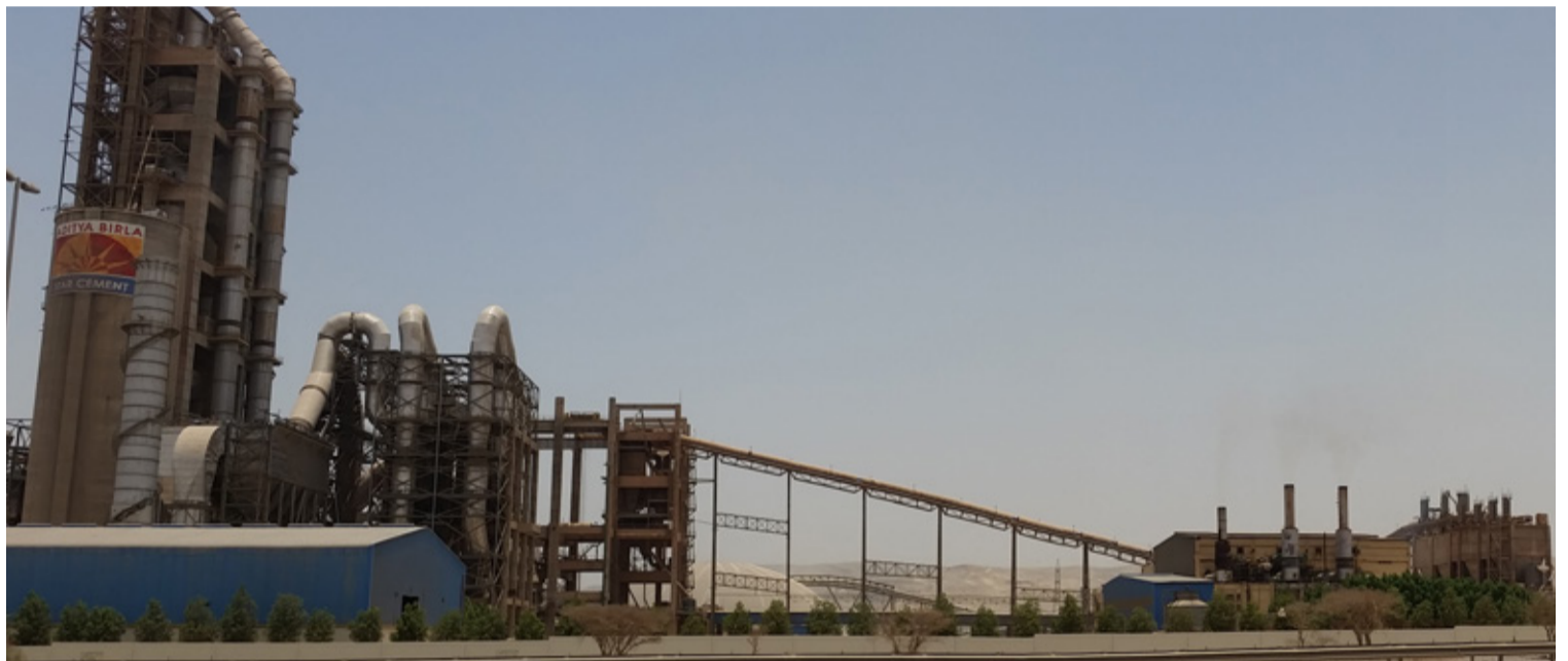
Star Cement Clinker plant in Ras al-Khaimah, which operates three MAN B&W 9L58/64 engines.
