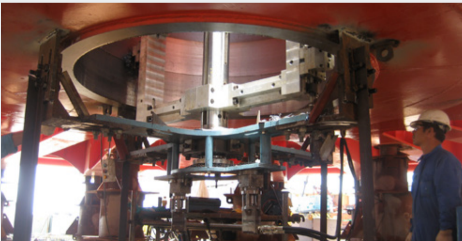
Goltens G2000 boring machine at work on the Leewek Constellation 's 2.1 meter diameter 400-ton deck reel hub bearing housings in Triyards shipyard in Vietnam.
