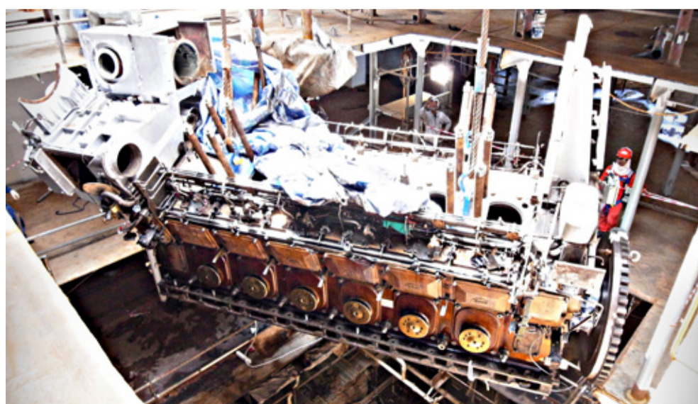
Rigging of the damaged MAN B&W 12V32/40 from the vessel for repairs.
