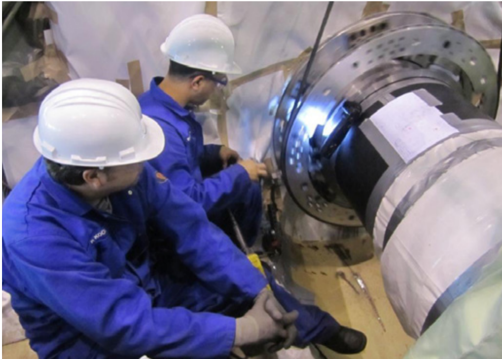
Goltens In-Situ machinists machining a 610mm diameter shaft on a newly installed Hitachi TC4F steam turbine journal that was damaged during operational testing at the Maasvlakte Electrabel Powerplant in the port of Rotterdam. Working closely with the manufacturer's technical representatives, Goltens removed 1.20mm from the shaft diameter and finished the journal surface to 0.12Ra.
