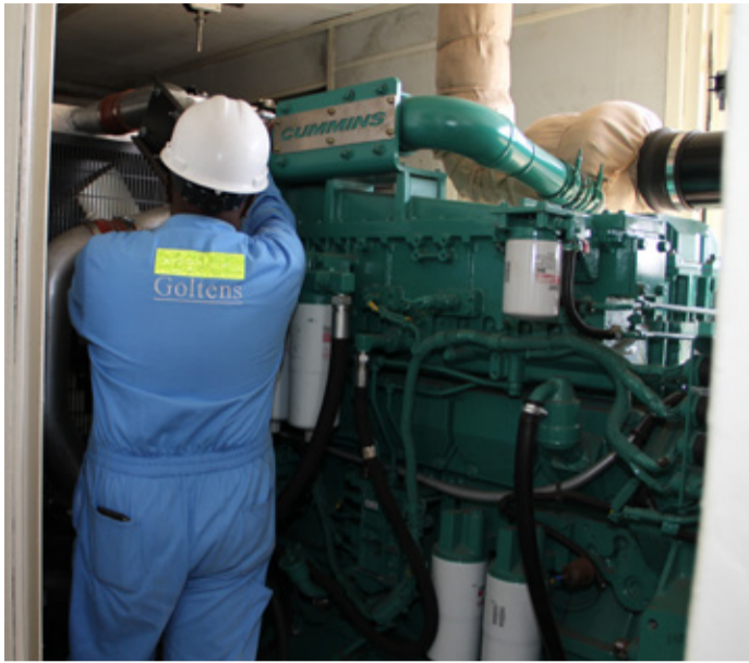
One of Goltens' specialist engineers working on one of the 18 Cummins Gensets.
