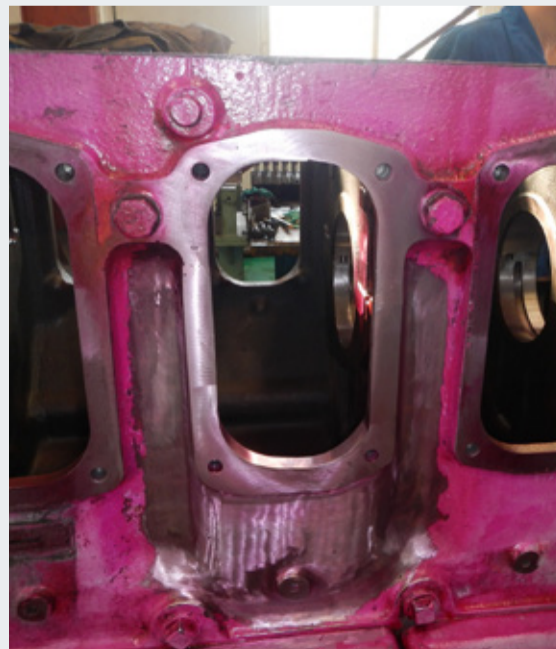
Dye penetrant crack check on the completed repair.
