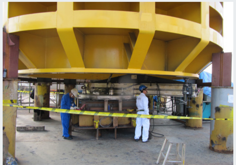
Flange facing of the underside of a turret head on an FPSO conversion project in Keppel Shipyard in Singapore (OD 5.99m/ID 5.58m)
