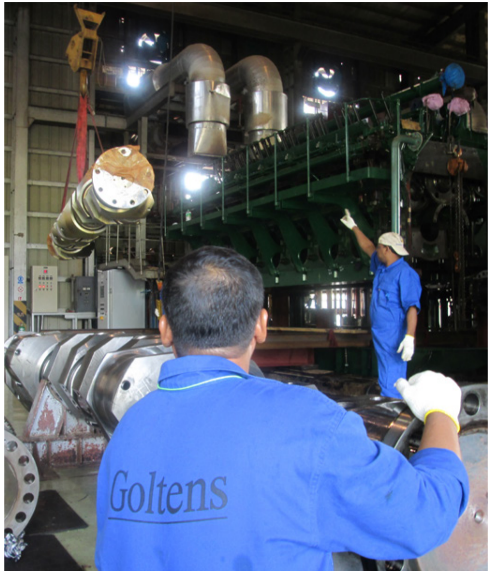
Goltens technicians rigging replacement Sulzer Z40/48 crankshaft into position at Tarlac Power.
