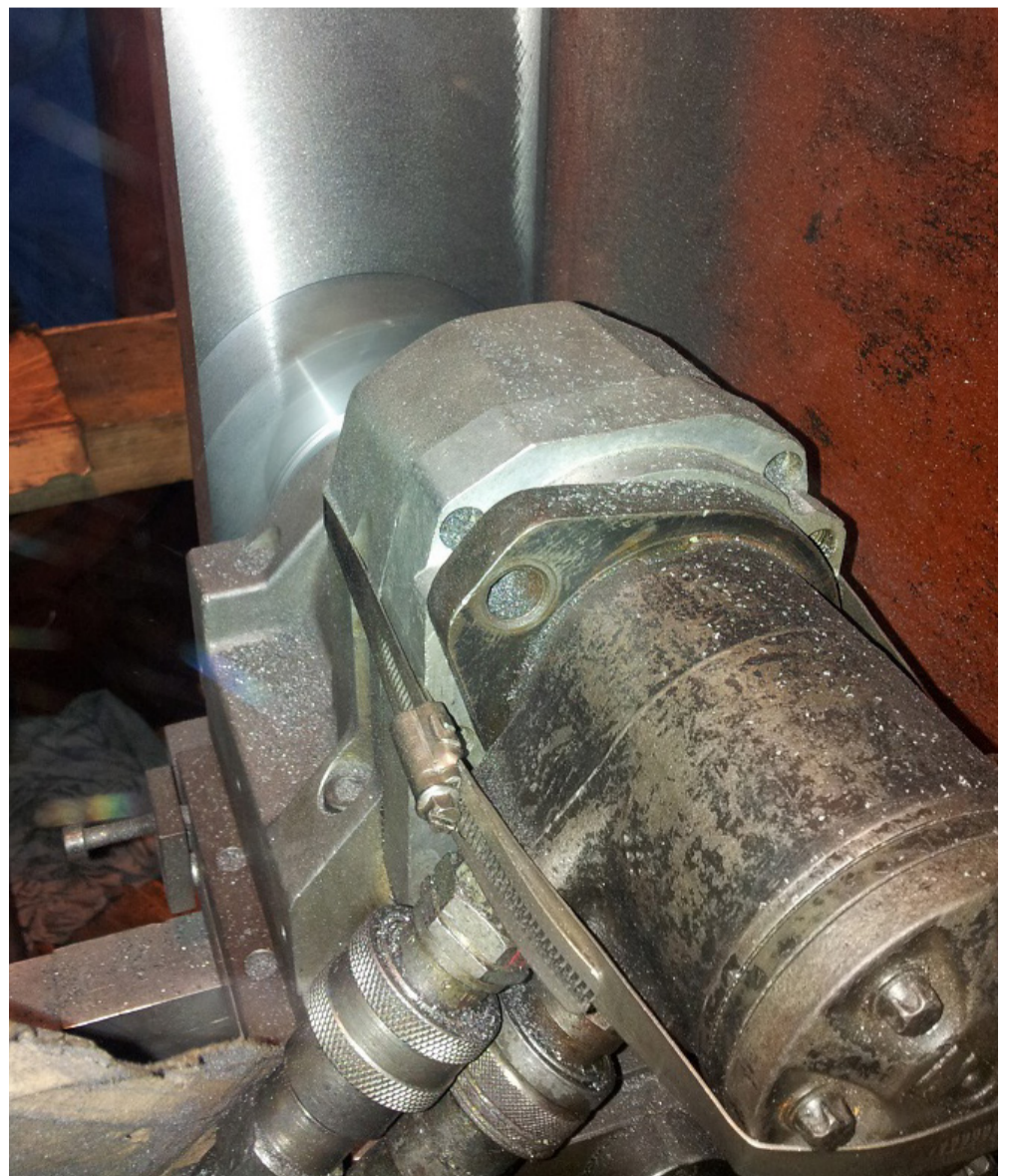
Machining near completion on one of the damaged guide rails. Deep scoring has been removed.
