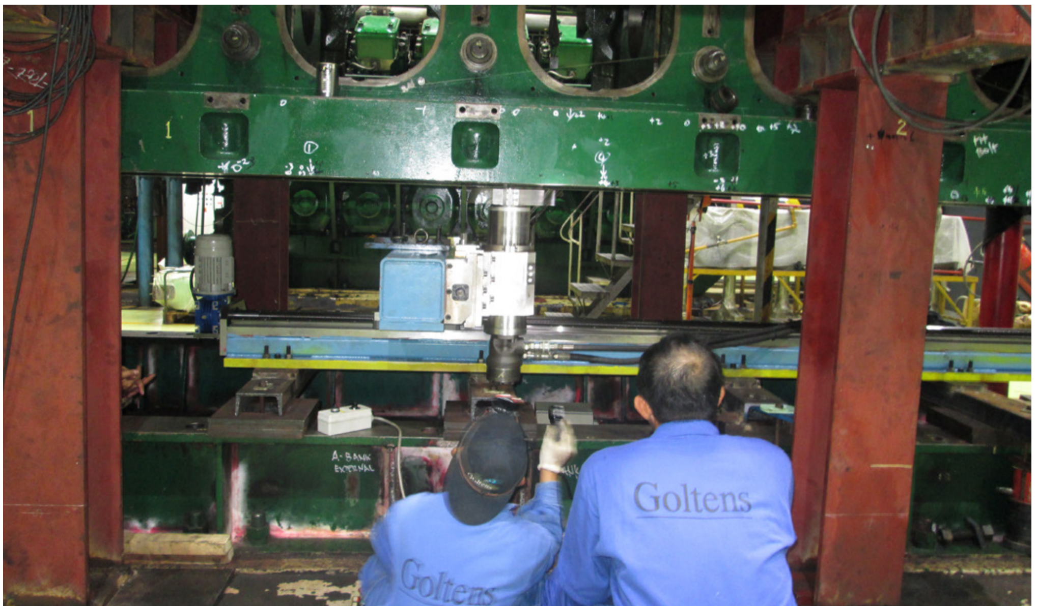
Goltens In-Situ machinists milling the underside mating surface of the Sulzer Z40/48 engine block to remove distortions.
