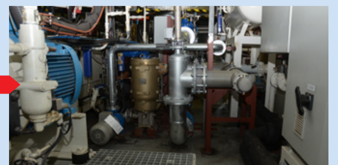
Installed Optimarin BWT system.
