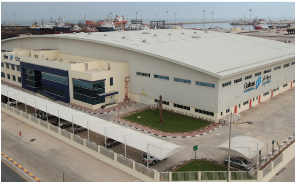
Goltens new facility in Dubai Maritime City includes 10,000 square meters of workshops, 1,500 square meters of offices, 10,000 square meters of open yard and a prime location abutting DMC's docking yard.
