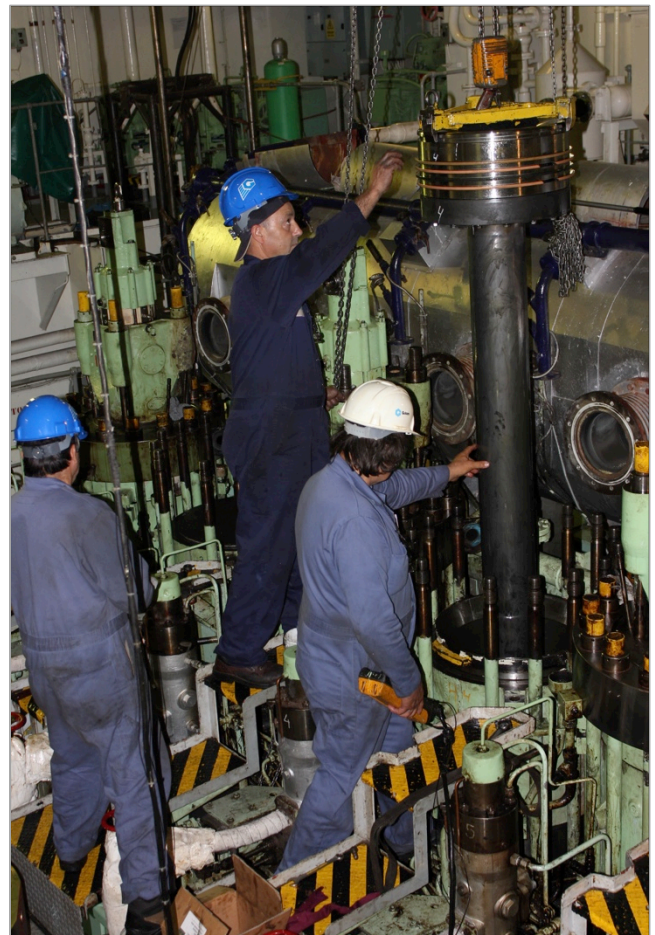
Goltens' technicians installing repaired piston
